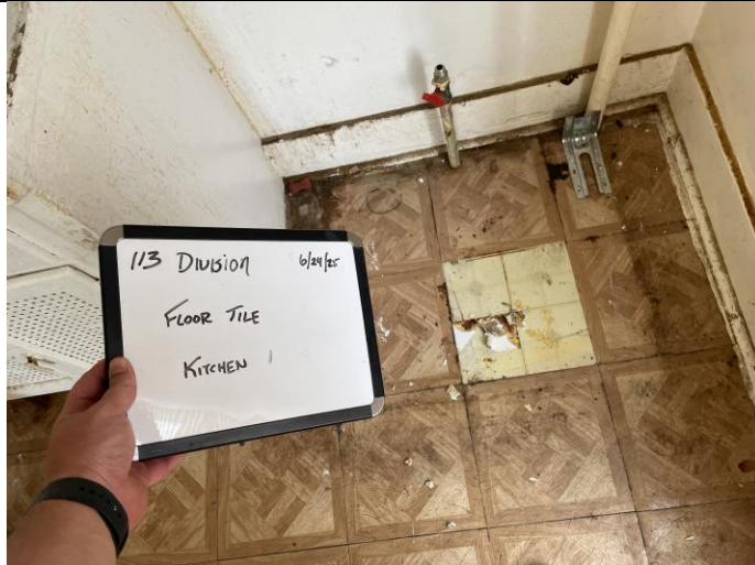
Date: 6/24/25 Location: Kitchen 1 Description: Floor Tile
